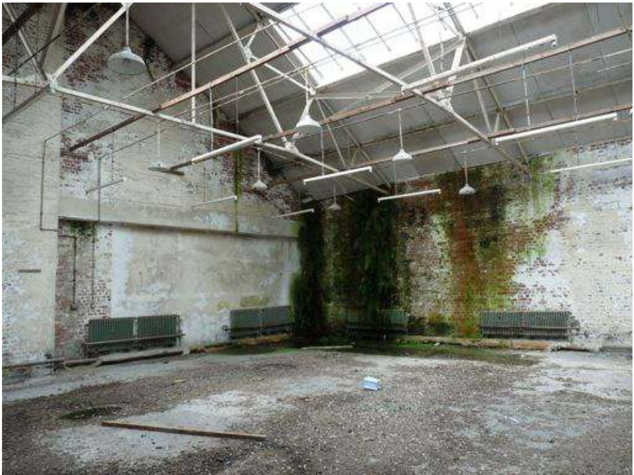
Image 6: Disused sorting office behind the old Post office
