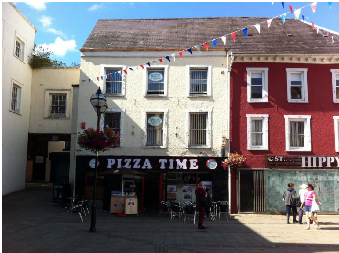
View 6: Buildings North side
